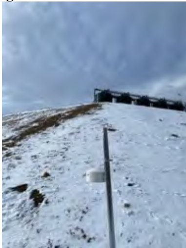
Looking towards the Site from the East
