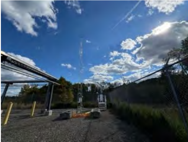
Looking towards the Site from the North
