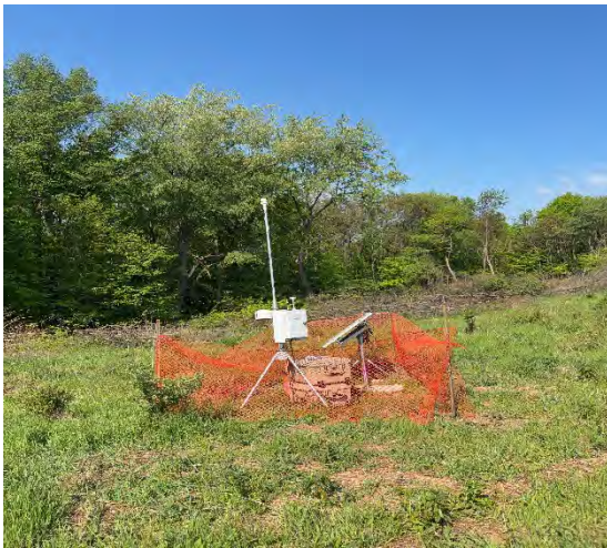
Looking towards the Site from the East
