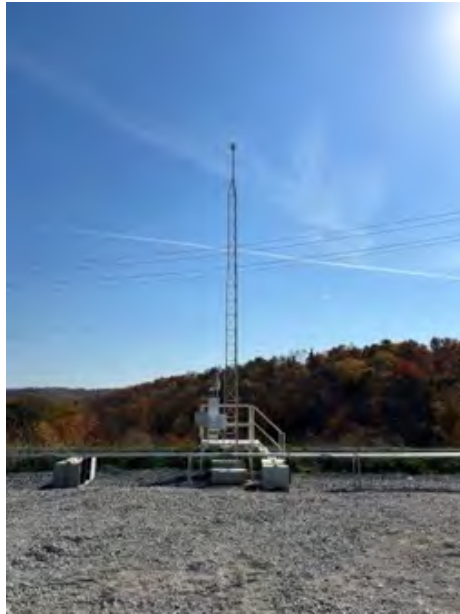
Looking towards the Site from the North
