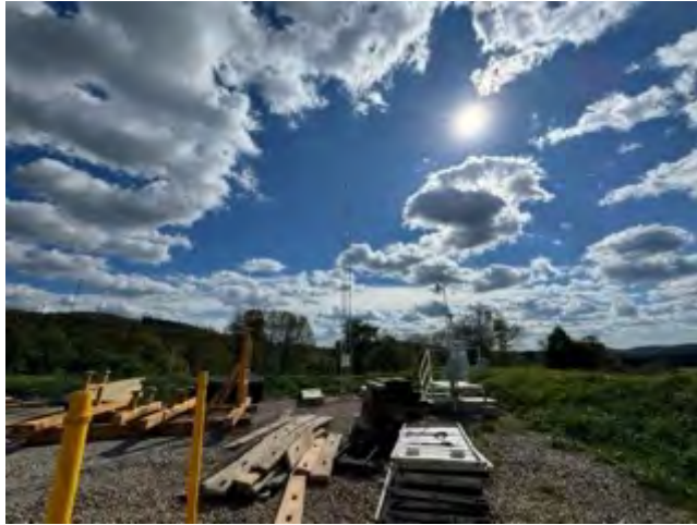
Looking towards the Site from the North
