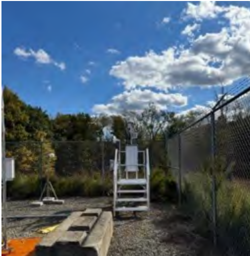
Looking towards the Site from the North
