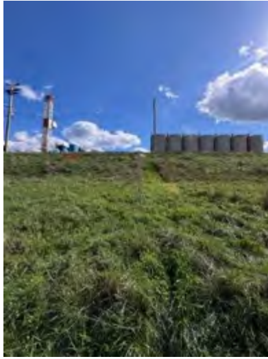
Looking towards the Site from the North
