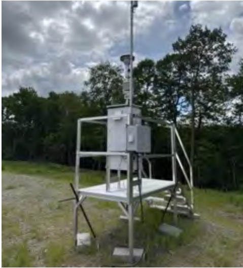
Looking towards the Site from the North
