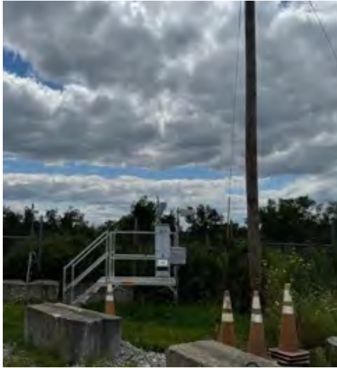
Looking towards the Site from the North
