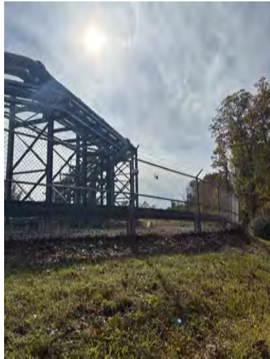
Looking towards the Site from the North
