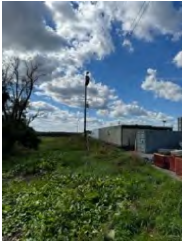
Looking towards the Site from the East
