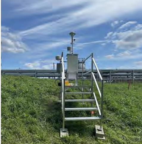
Looking Towards the Site from the North
