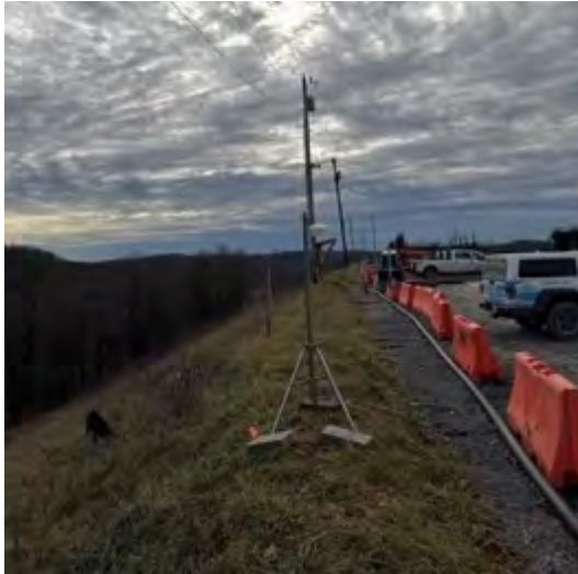
Looking towards the Site from the North
