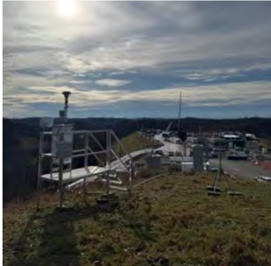
Looking towards the Site from the North
