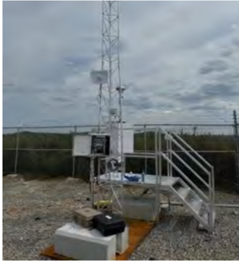
Looking towards the Site from the North
