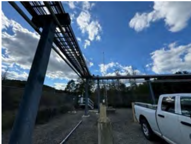
Looking towards the Site from the East
