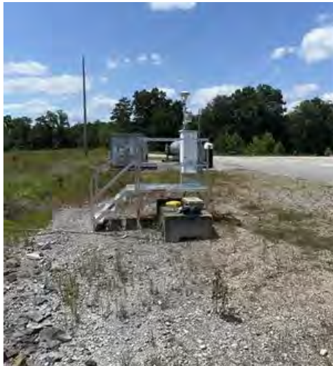
Looking towards the Site from the East
