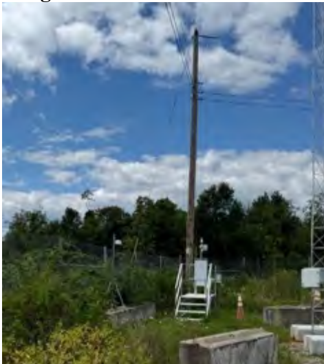
Looking towards the Site from the East
