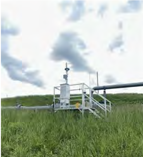
Looking towards the Site from the North
