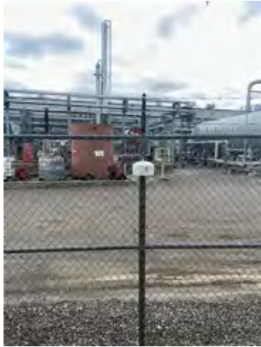
Looking towards the Site from the North
