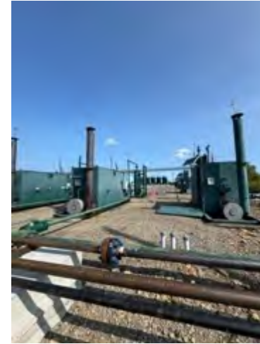
Looking towards the Site from the South*
