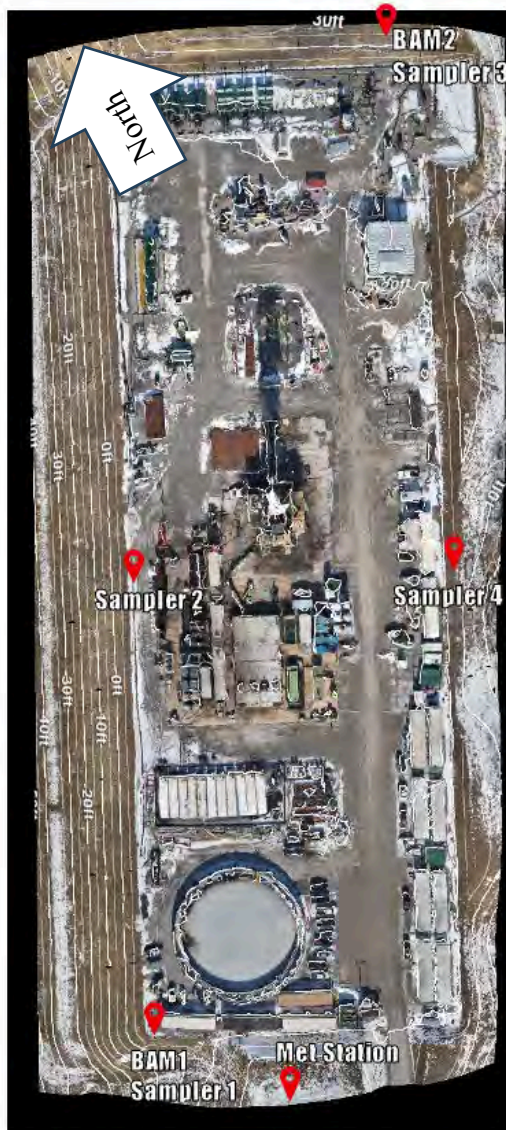
Figure AG-1. Aerial View of the WDTN18 Well Pad and Monitoring Locations (BAM-1 and BAM-2: PM2.5 Monitors, Met Station: Meteorological Measurement System, Sampler 1 – 4: Passive BTEX Sampling Location). Contour Lines Represent a 5 ft Elevation Difference. Note: While all monitoring locations are depicted, markers may not be precise due to space limitations of the aerial image.
