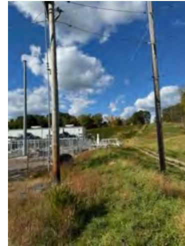
Looking towards the Site from the South*
