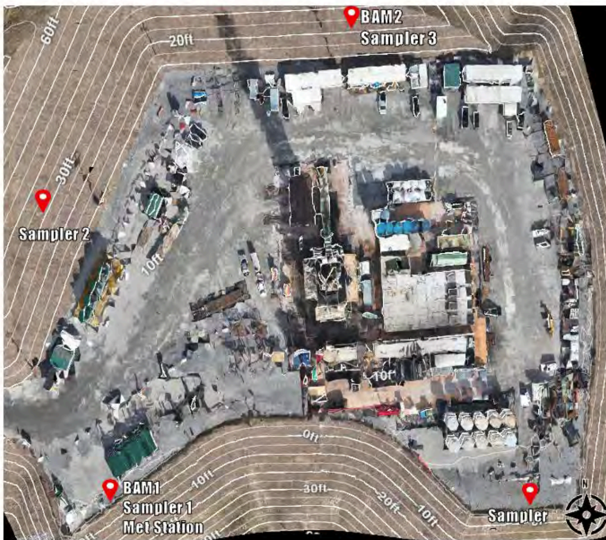
Figure AN-1. Aerial View of the WFN12 Well Pad and Monitoring Locations (BAM-1 and BAM-2: PM2.5 Monitors, Met Station: Meteorological Measurement System, Sampler 1 – 4: Passive BTEX Sampling Location). Contour Lines Represent a 5 ft Elevation Difference.
