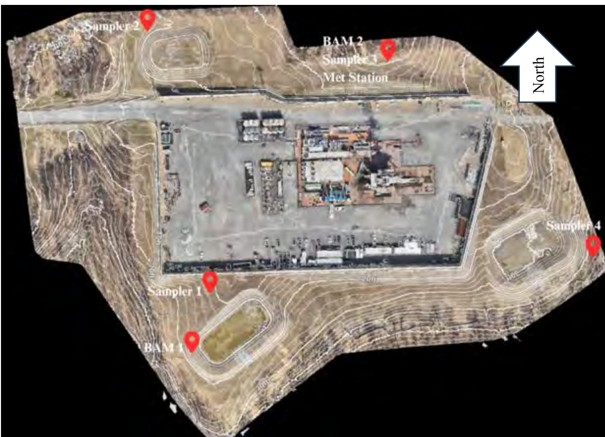
Figure AS-1. Aerial View of the MAM14 Well Pad and Monitoring Locations (BAM-1 and BAM-2: PM2.5 Monitors, Met Station: Meteorological Measurement System, Sampler 1 – 4: Passive BTEX Sampling Location). Contour Lines Represent a 2 ft Elevation Difference.
