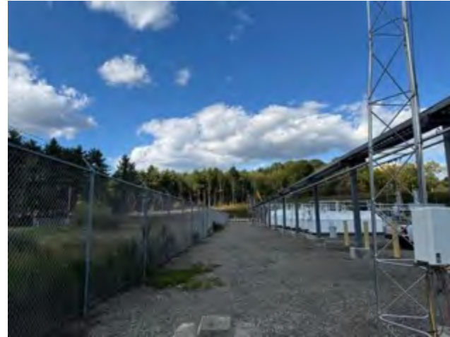
Looking towards the Site from the South*
