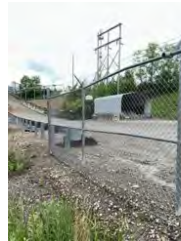
Looking towards the Site from the South
