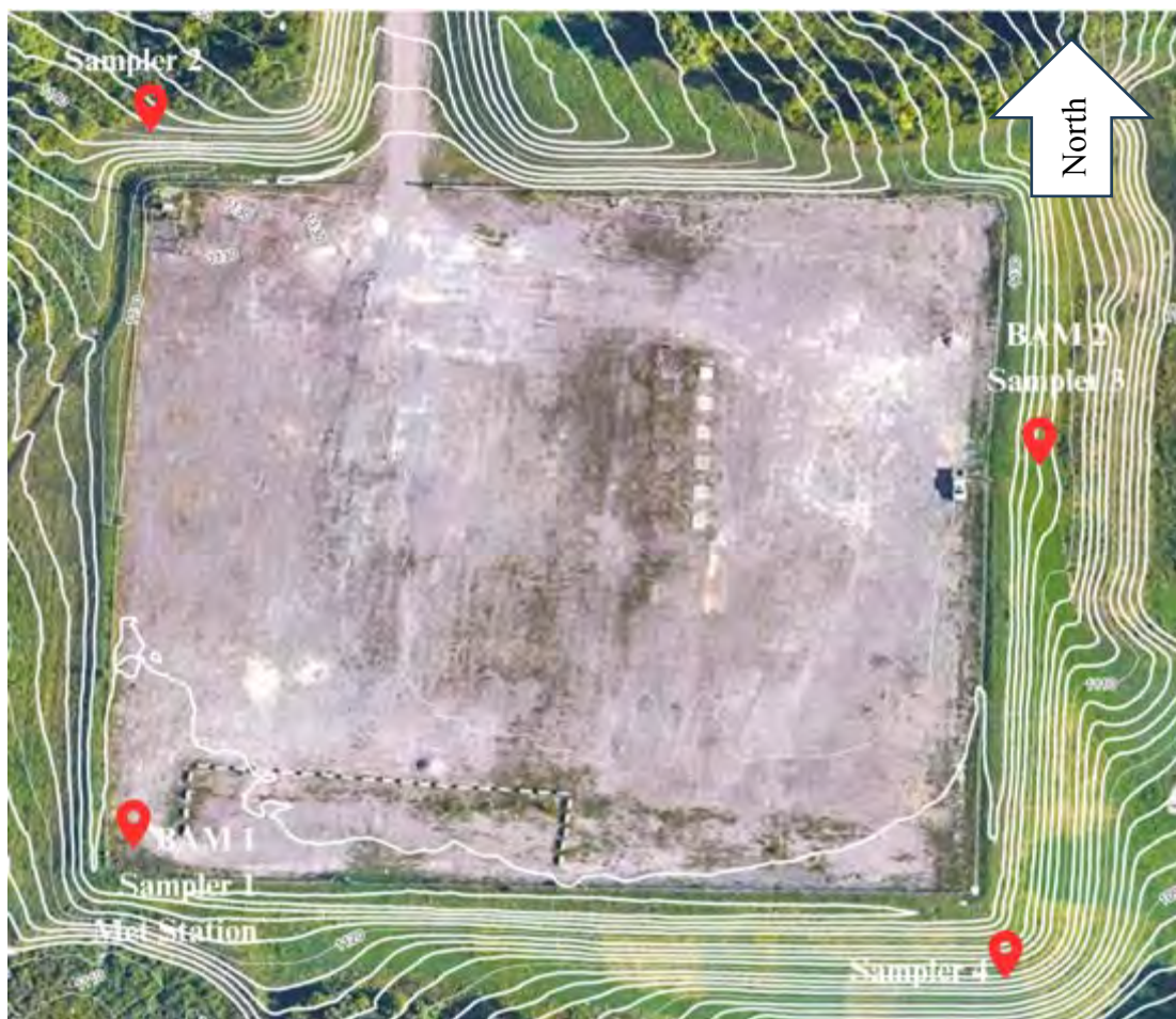
Figure AF-1. Aerial View of the ACAA4 Well Pad and Monitoring Locations (BAM-1 and BAM-2: PM 2.5 Monitors, Met Station: Meteorological Measurement System, Sampler 1 – 4: Passive BTEX Sampling Location). Contour Lines Represent a 2 ft Elevation Difference. Note: Topography may not be fully up to date due to restrictions on drone photography near the airport.
