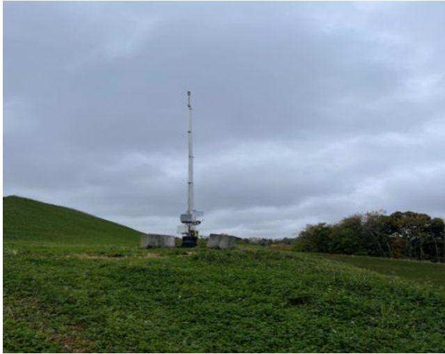
Looking towards the Site from the North
